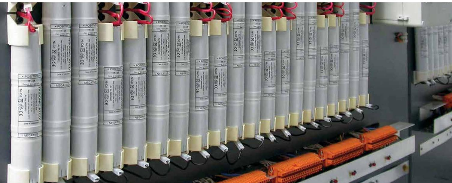
Emergency lighting is a safety-relevant issue and, because of this, there are strict standards to adhere to, of which the most relevant are the luminaire standard IEC 60598-2-22 and the component standard for self-contained emergency lighting IEC 61347-2-7. Differences in the performance of batteries are not only due to different battery chemistries, but stem from differences in the quality of each individual cell.
